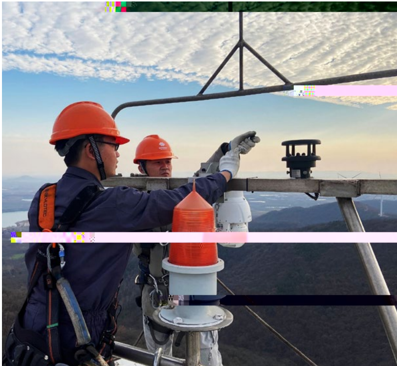
Employees set up full-vision camera outside the cabin
